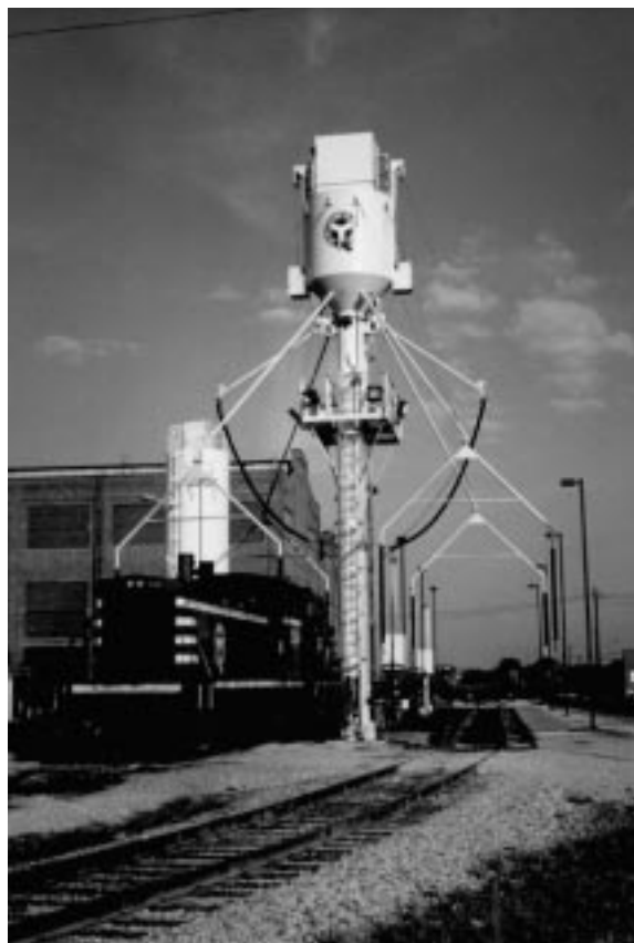
The Belt Railway's modernized locomotive service facility can provide fuel, water, lube oil, and sand to six locomotives at one time. The facility now handles 1,600 to 1,800 locomotives per month.
