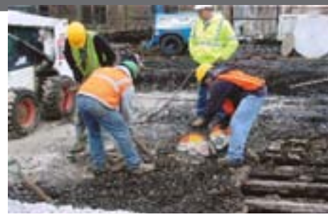
BRC employees replace the 80th Street bridge concrete deck with a steel plate.
