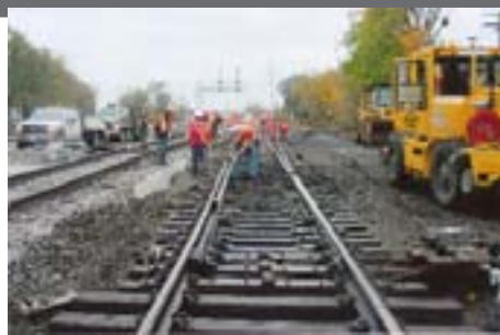
BRC employees replace the 80th Street bridge concrete deck with a steel plate.
